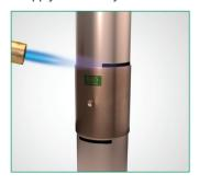
Apply heat, keeping the flame moving to ensure that parent metals are evenly heated to a cherry-red color.
