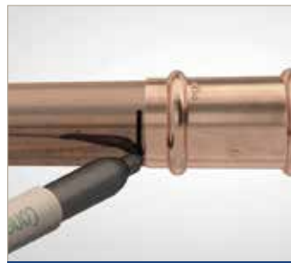
6. Assemble and mark the insertion depth
