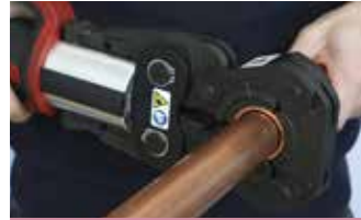
3. Complete the joint with the press tool
