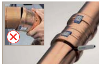
6. Mark the insertion depth
