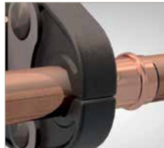
7. Complete the joint with the press tool
