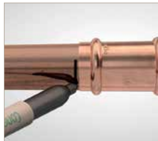
6. Assemble and mark the insertion depth
