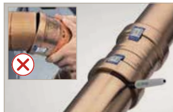
6. Mark the insertion depth
