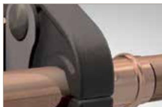
7. Complete the joint with the press tool
