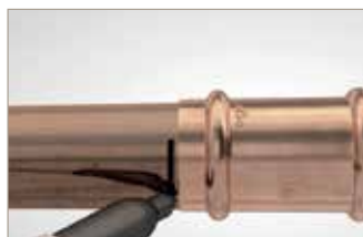
6. Assemble and mark the insertion depth
