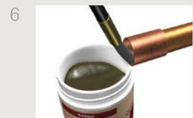
6 Apply flux to the inside of the socket
